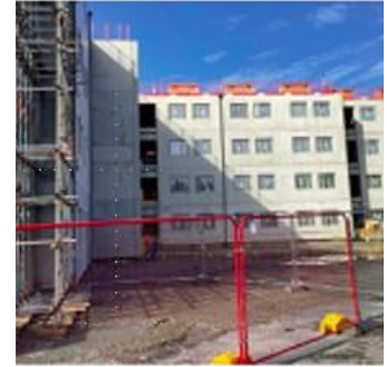
Accelerated House Blocks
